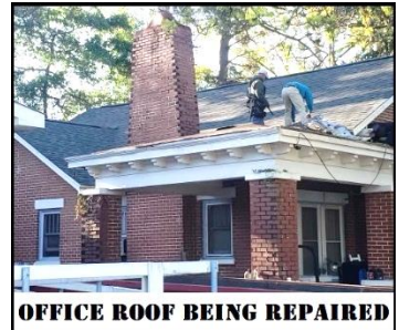
OFFICE ROOF BEING REPAIRED
