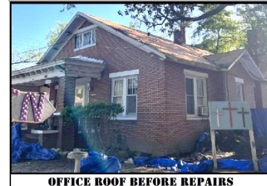
OFFICE ROOF BEFORE REPAIRS
