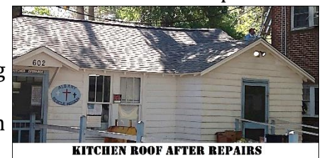
KITCHEN ROOF AFTER REPAIRS
